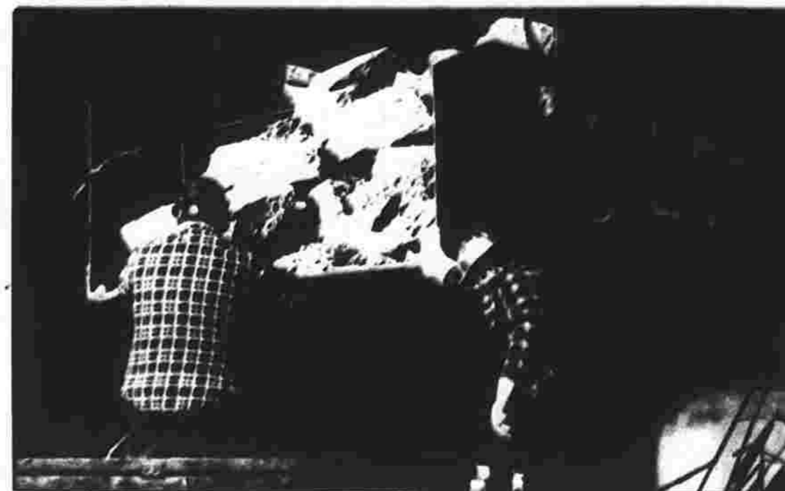
Workers guide a load of concrete onto a truck Friday at the site of the apartment building collapse in Bridgeport as the rescue effort continues.
